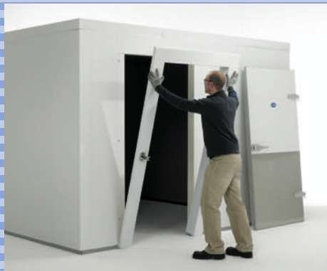
1. Set the new replacement frame in place.
