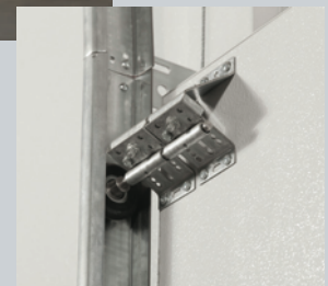
Vertical track with roller
