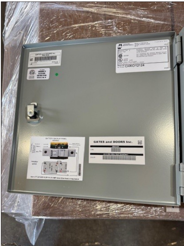
Figure 9-4. BATTERY BACKUP DOOR OPERATOR NEMA4 ENC_
