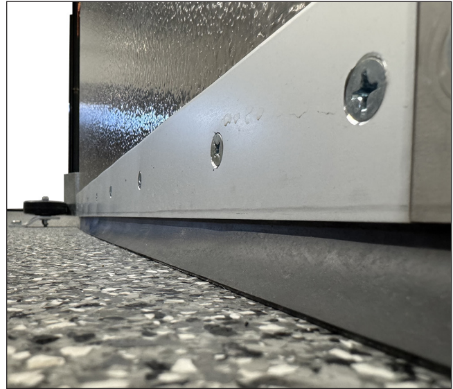
Figure 4-9. Bottom Seal
